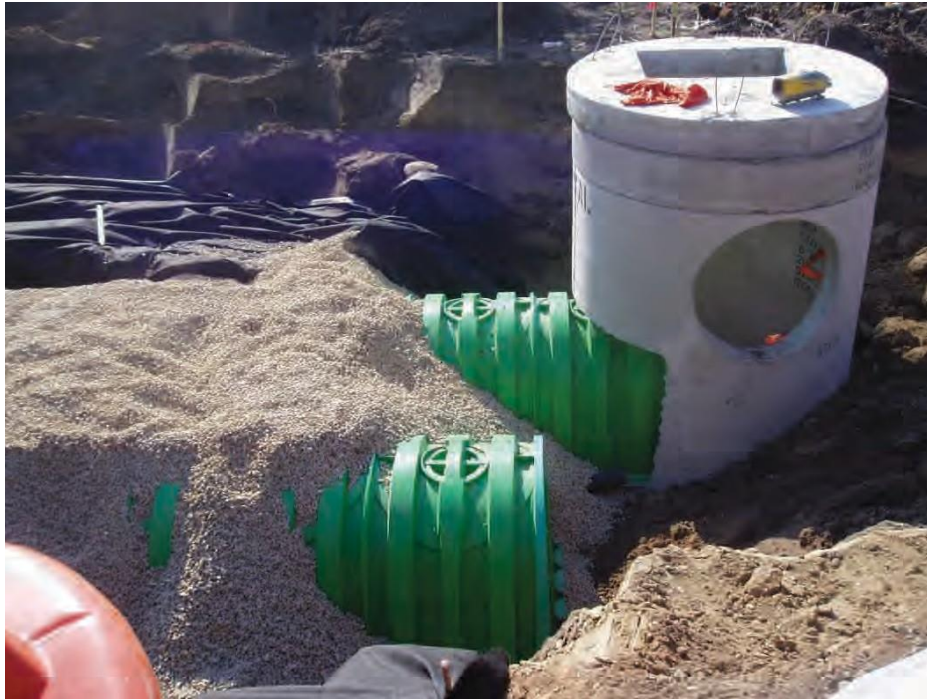
Figure 6 - Chamber direct connection option
